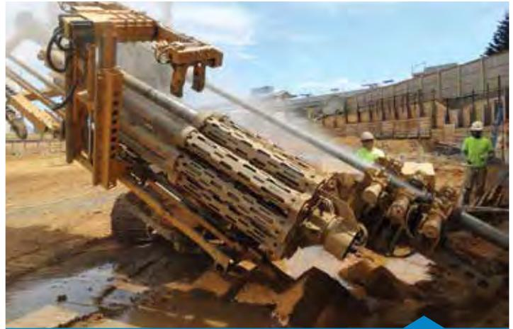
BERKEL FACED STUBBORN QUARTZITE ON THE SOUTH SIDE OF THE SITE, ALTHOUGH OVERALL DRILLING CONDITIONS WERE IDEAL BECAUSE MOST OF THE SITE CONSISTED OF SANDY CLAY AND PARTIALLY WEATHERED ROCK (PWR)
