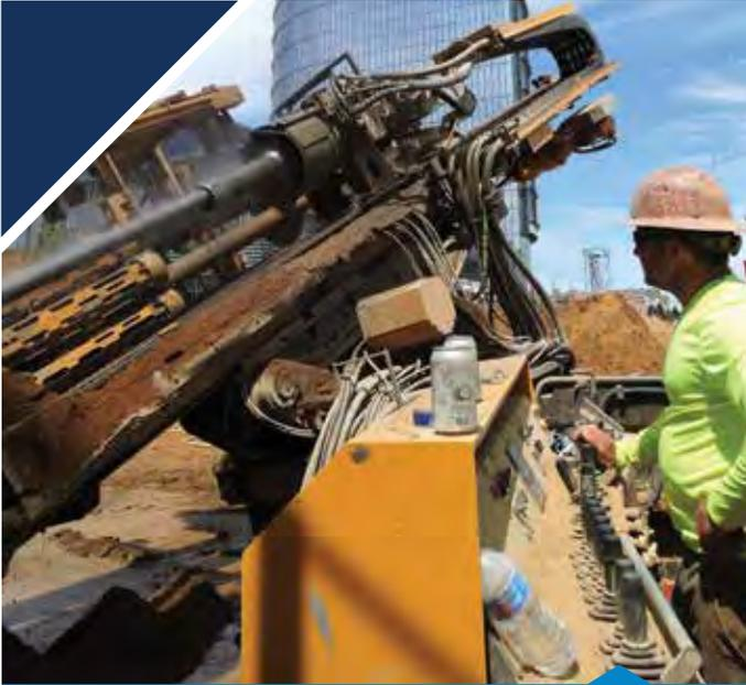
**BERKEL & COMPANY CONTRACTORS USED A KLEMM KR 807-7G DRILLING RIG TO INSTALL NEARLY 400 GROUTED TIEBACK ANCHORS TO HOLD UP THE SHORING WALLS OF A 50-FOOT CUT FROM GROUND LEVEL ON A MIXED-USE DEVELOPMENT IN TYSONS CORNER, VA**
