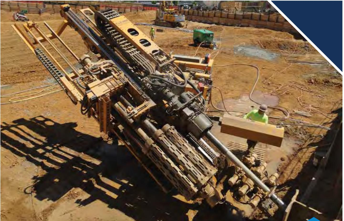
THE KR 807-7G INSTALLED SIX-INCH DIAMETER TIEBACK ANCHORS TO DEPTHS RANGING FROM 65 TO 75 FEET
