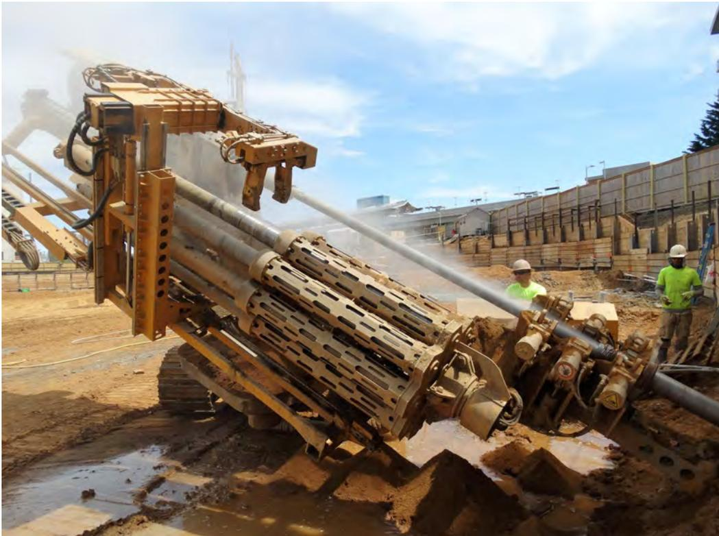
*Berkel faced stubborn Quartzite on the south side of the site, although overall drilling conditions were ideal because most of the site consisted of sandy clay and Partially Weathered Rock (PWR).*
