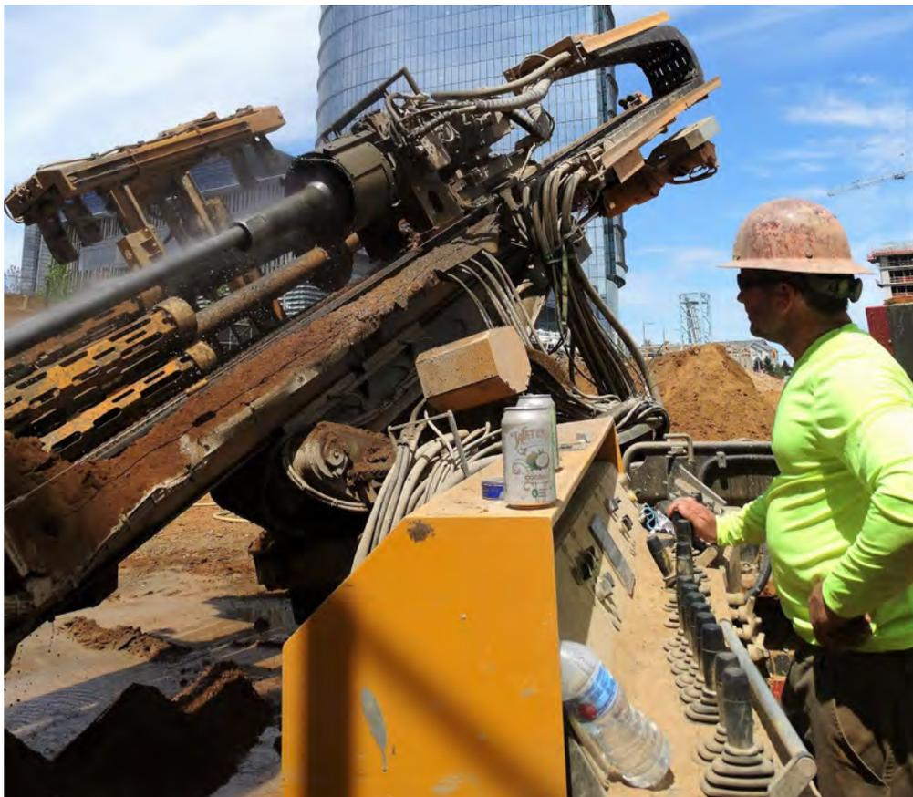
*Berkel & Company Contractors used a KLEMM KR 807-7G Drilling Rig to install nearly 400 grouted tieback anchors to hold up the shoring walls of a 50-foot cut from ground level on a mixed-use development in Tysons Corner, Va.*
