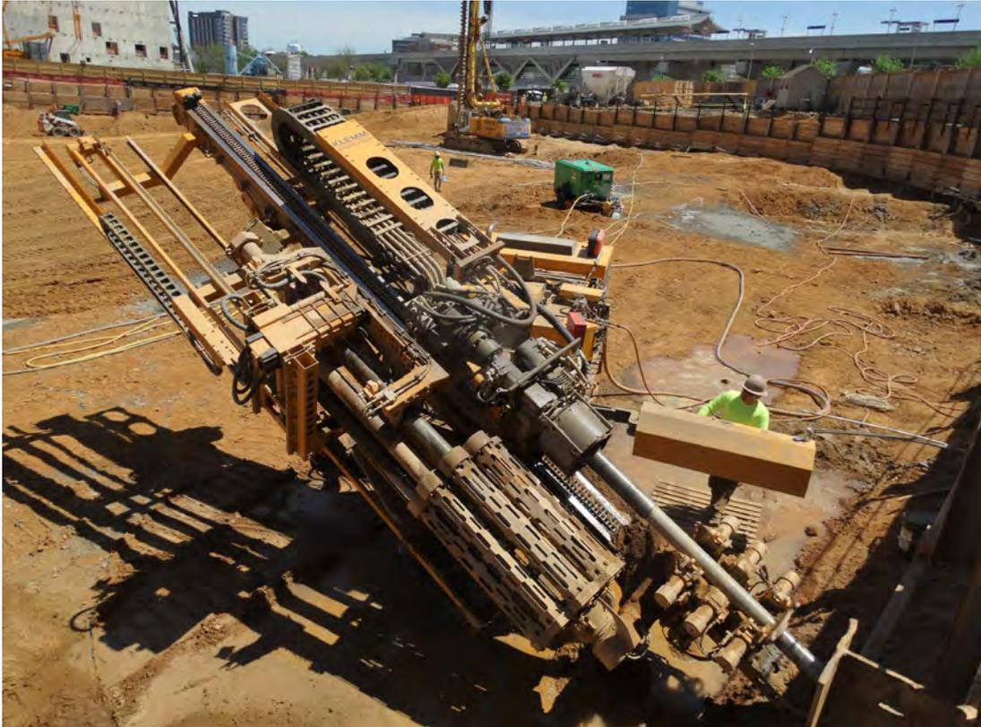
*The KR 807-7G installed six-inch diameter tieback anchors to depths ranging from 65 to 75 feet.*
